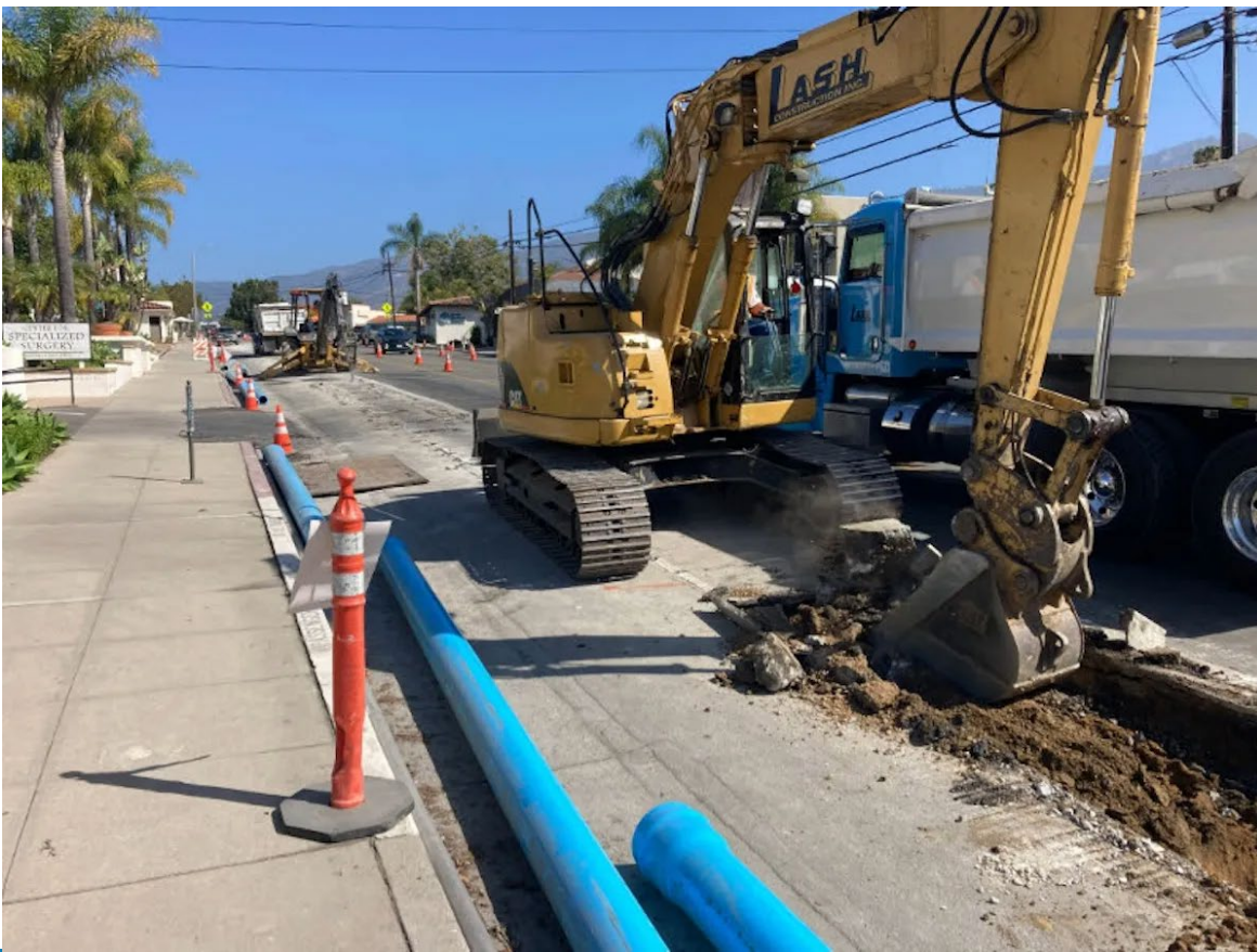
Street Pipeline Construction (2028)
