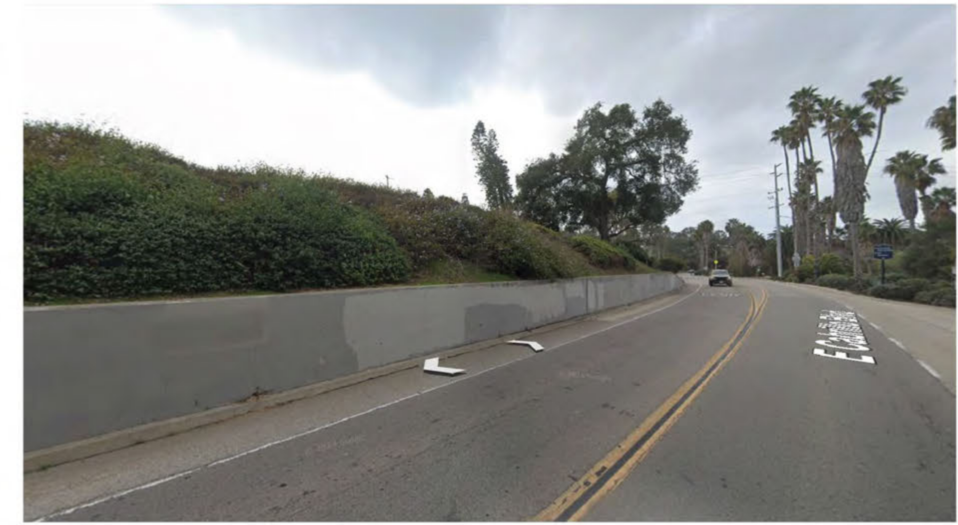
View from E.Cabrillo towards South West (1)
