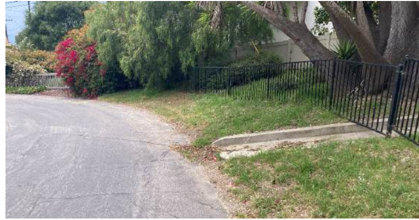
Photograph 10. Pedestrian view of proposed relining exit pit area on La Vista Del Oceano, facing south ( Exit Pit for La Vista Del Oceano Pipeline Lining ).
