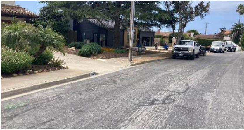
Photograph 9. Pedestrian view of lining entry pit area on Ricardo Avenue, facing south ( Entry Pit for La Vista Del Oceano Pipeline Lining ).
