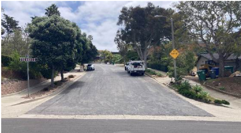
Photo 10. Pedestrian view of Ricardo Avenue at Dolores Drive, facing southeast ( New Ricardo Main ).
