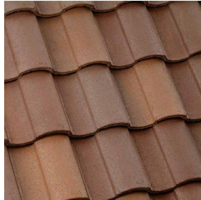
2. CONCRETE TILE ROOF
