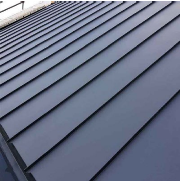
6. STANDING SEAM ROOF
