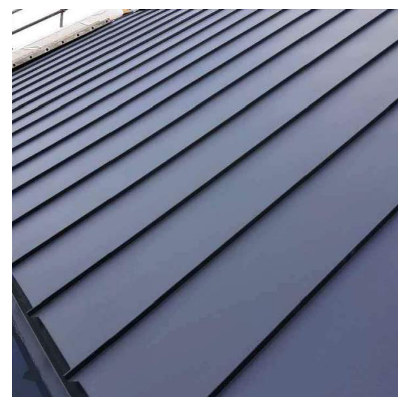
6. STANDING SEAM ROOF
