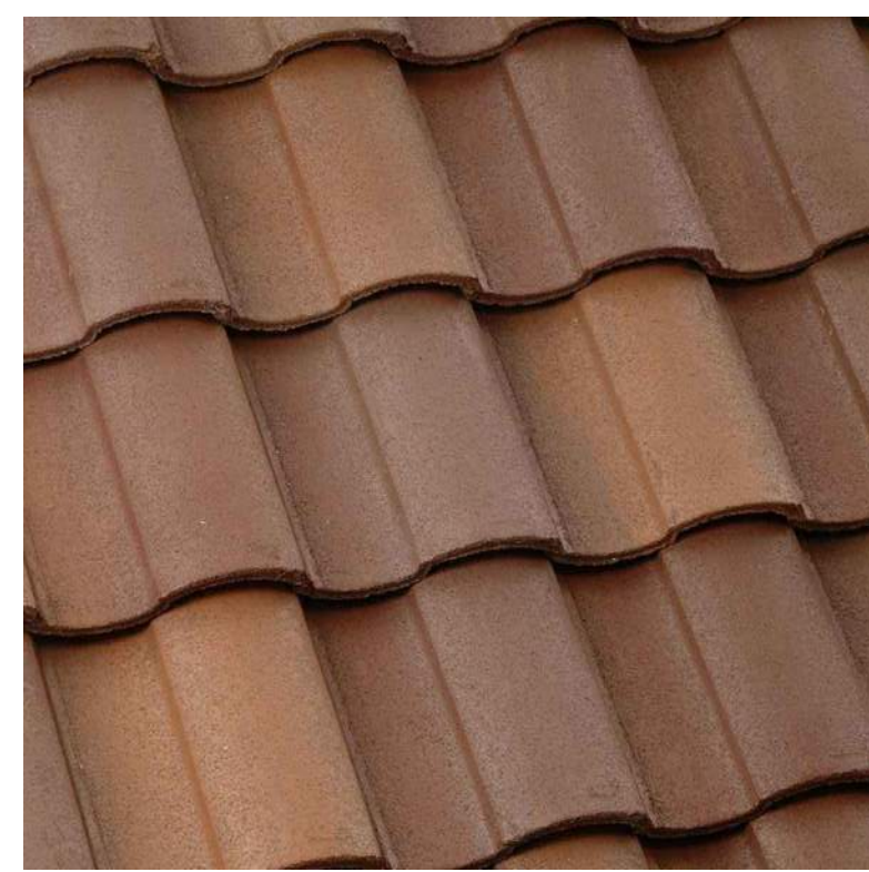
2. CONCRETE TILE ROOF
