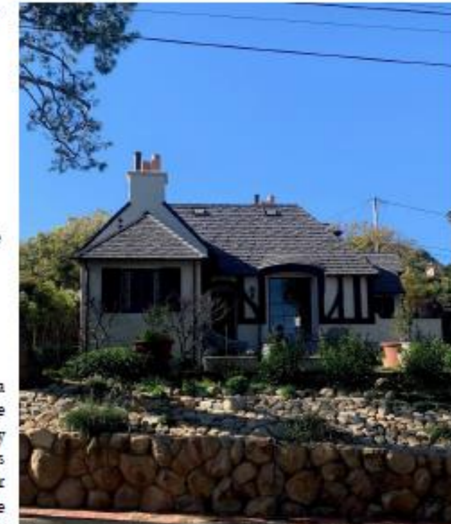
826 Coronel Street with steeply pitched roof, decorative half-timbering, and a stucco chimney with multiple flues; all of which are character defining features of the Tudor Revival style. Photograph by Heidi Reidel, February 28, 2024.
