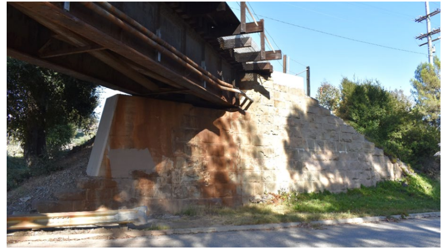
Photograph 2. Eastern sandstone abutment, looking east
