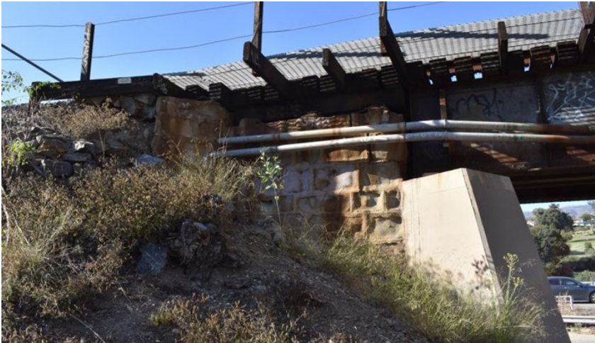
Photograph 1. Western abutment, looking northwest
