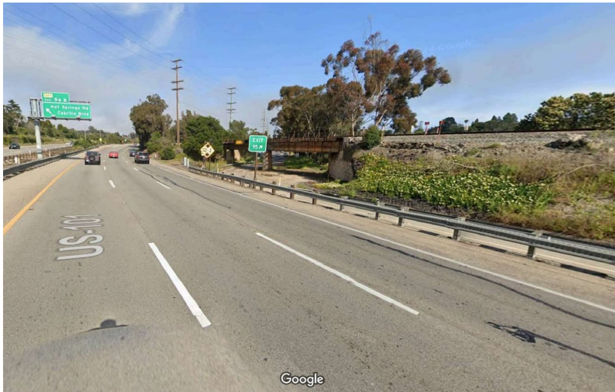
Figure 4.1-1 View of Project Site from U.S. 101
