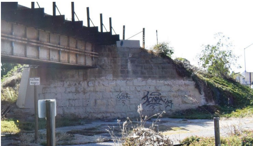
Photograph 3. Western sandstone abutment, looking west
