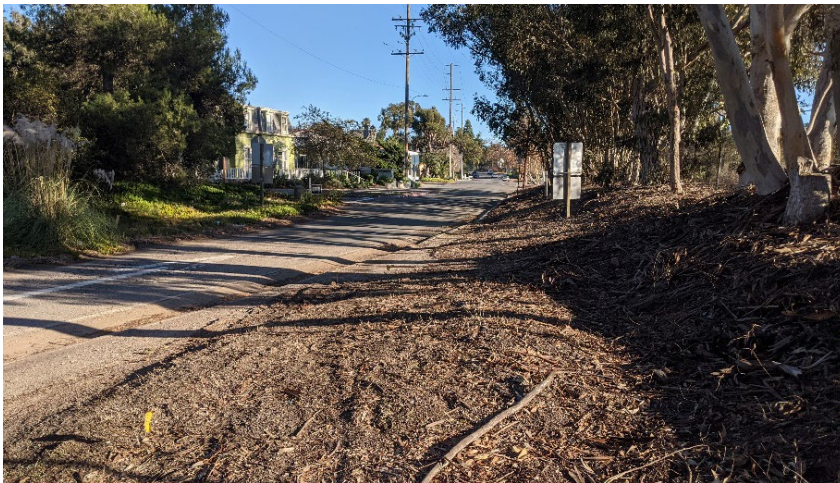
Photograph 3. View along Los Patos Way from off-ramp, facing southeast
