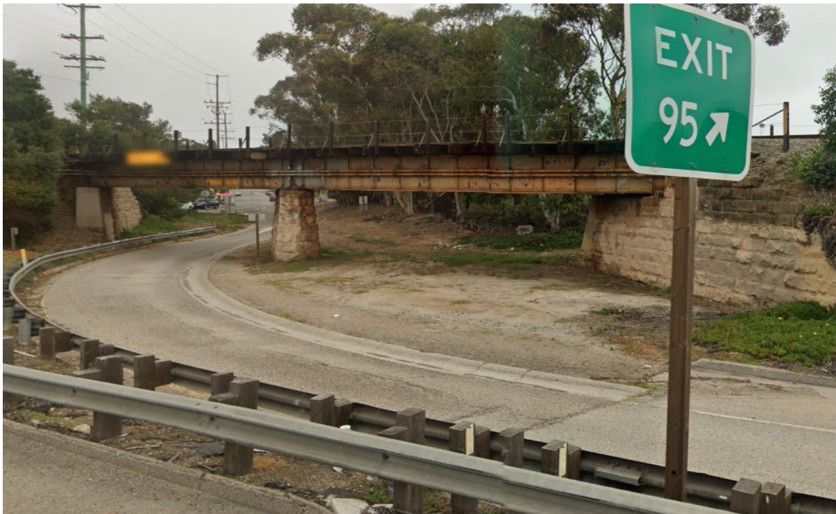
The Los Patos Way off-ramp and rail bridge, as seen from U.S. 101 north of the UPRR tracks, facing southeast.
