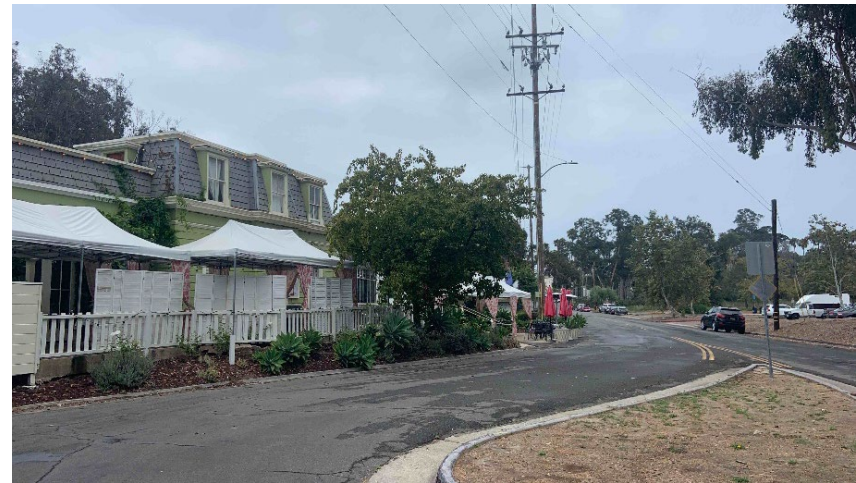
Photograph 4. View of development along Los Patos Way, facing northeast
