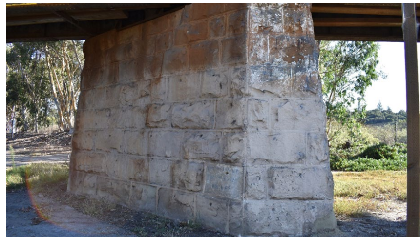
Photograph 4. Center sandstone pier, looking south
