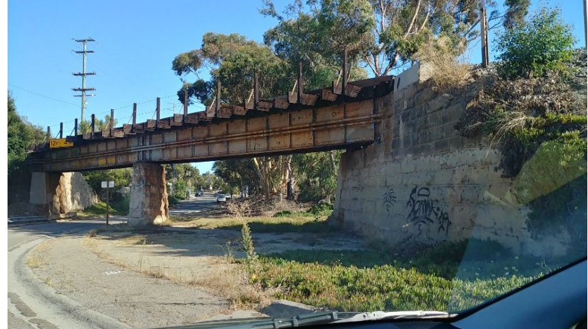
Photograph 2. View from Los Patos Way off-ramp, facing southeast
