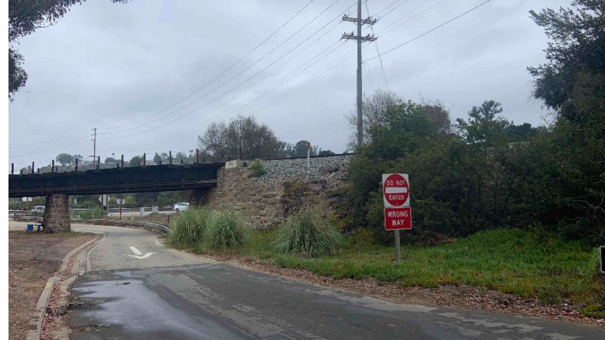
Photograph 2. Los Patos Rail Bridge, facing northwest
