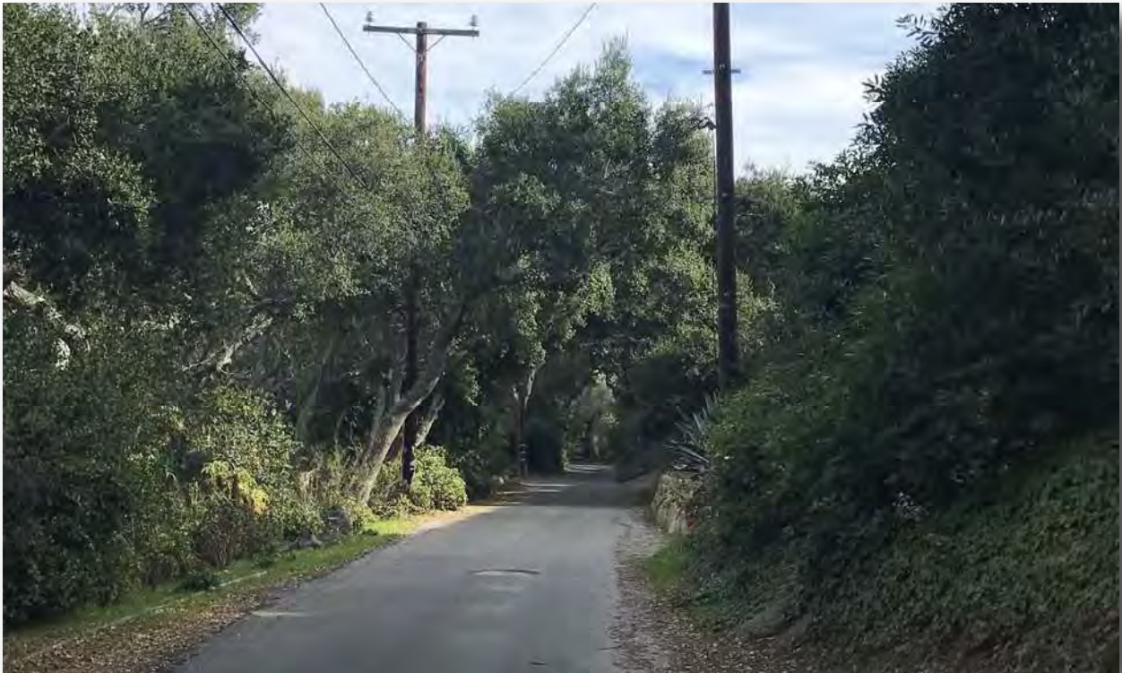
Photo F: View looking east along a local road within a High Fire Hazard Area and Vegetation Management Unit.
