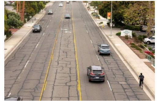
Existing Conditions along Cliff Drive
