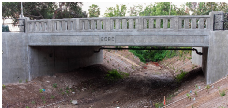
Quinientos St Bridge Replacement, Completed in 2020
