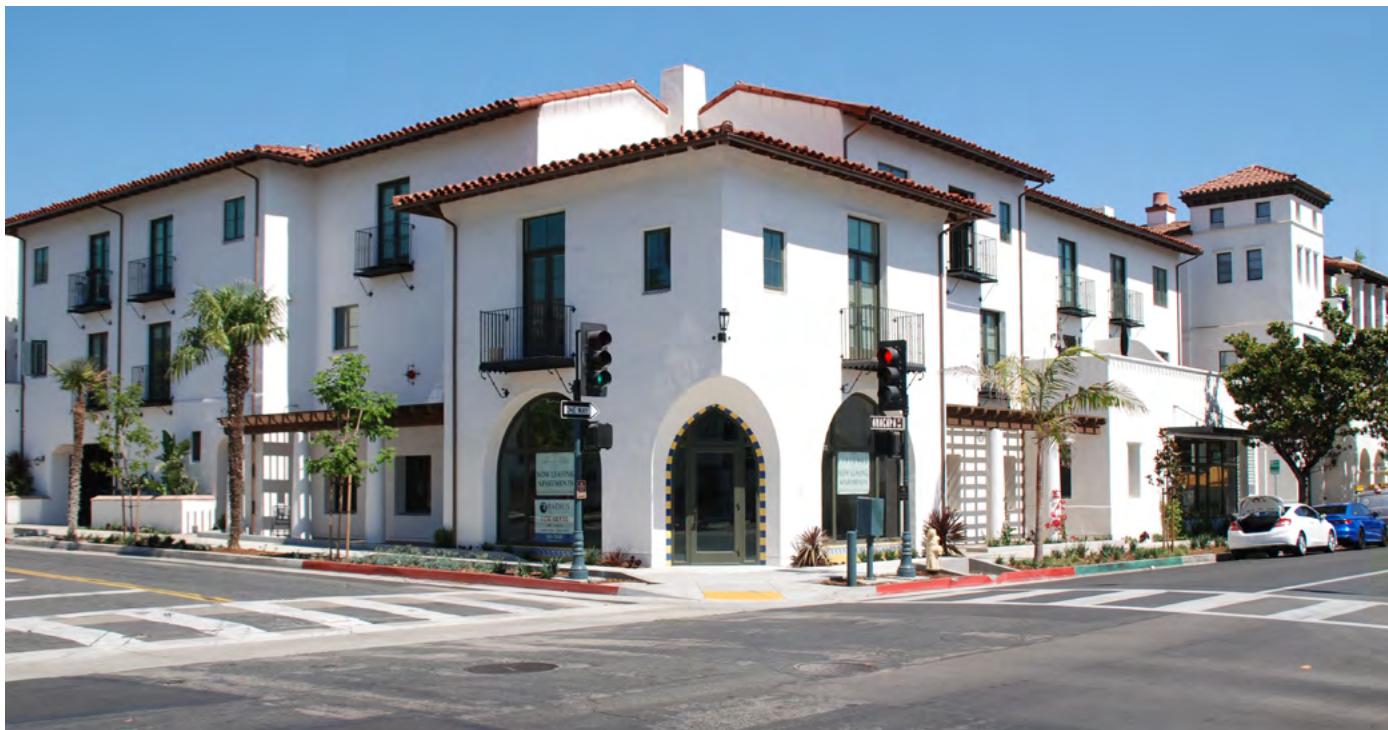
Local example in the Lower State neighborhood
