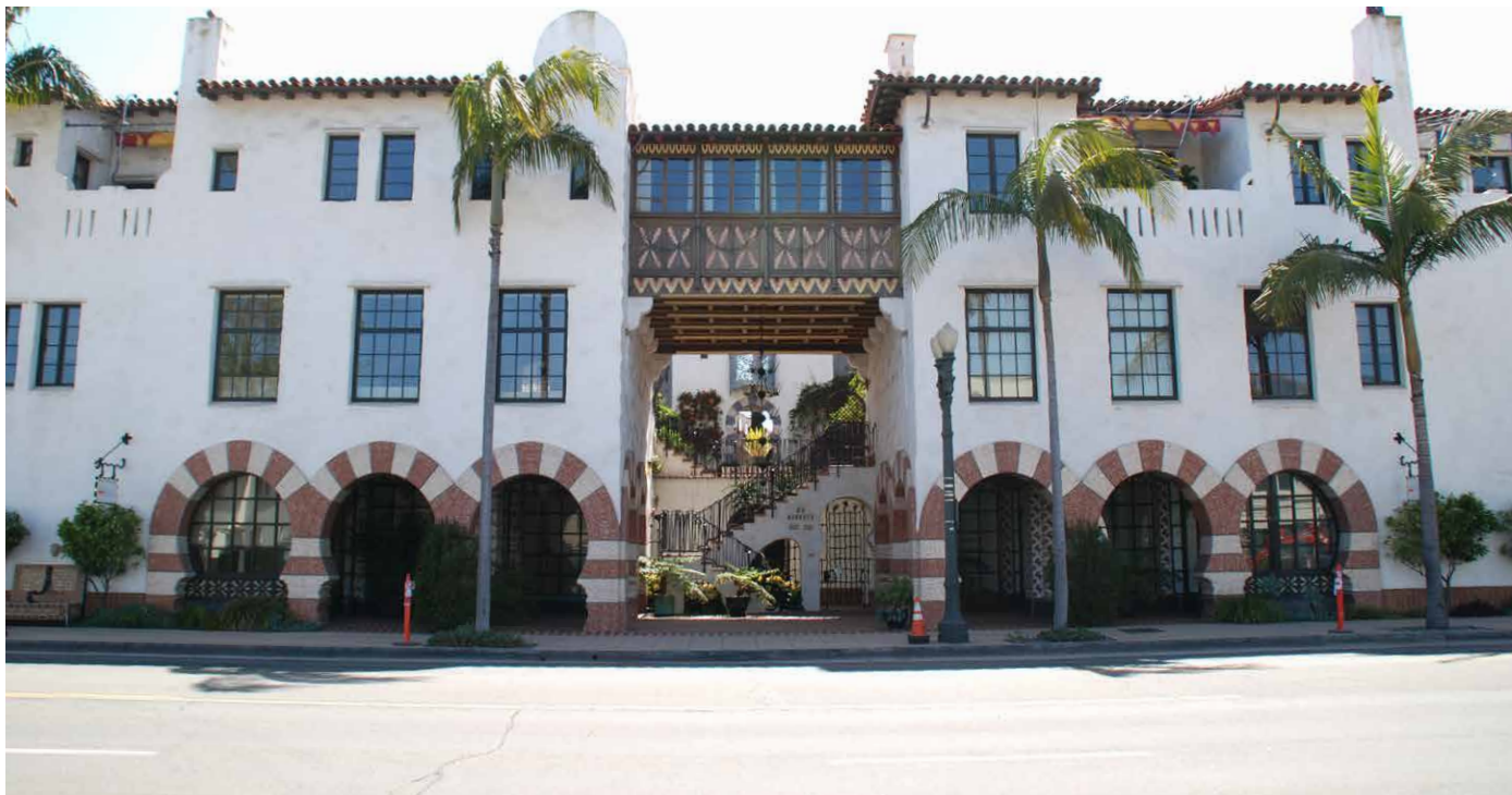
Local example in the West Downtown neighborhood
