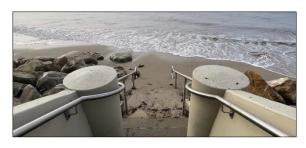
to extend the stairway below the wintertime scoured beach condition. The repairs include the installation of new handrails from the street level to the beach, construction of a new concrete guard-rail at the main landing mid-stairway, installation of a drain to capture groundwater to reduce algae growth and potentially slippery stair treads and re-pouring the concrete at the main landing to create positive drainage to the new drain.
