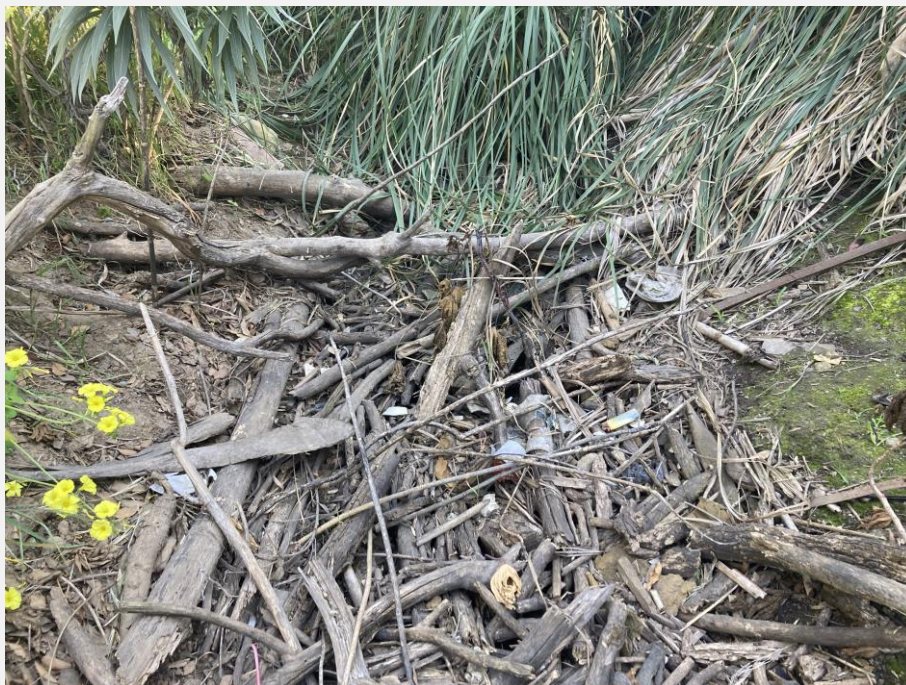
Photo 5. Debris within the storm drain ditch, March 3, 2022
