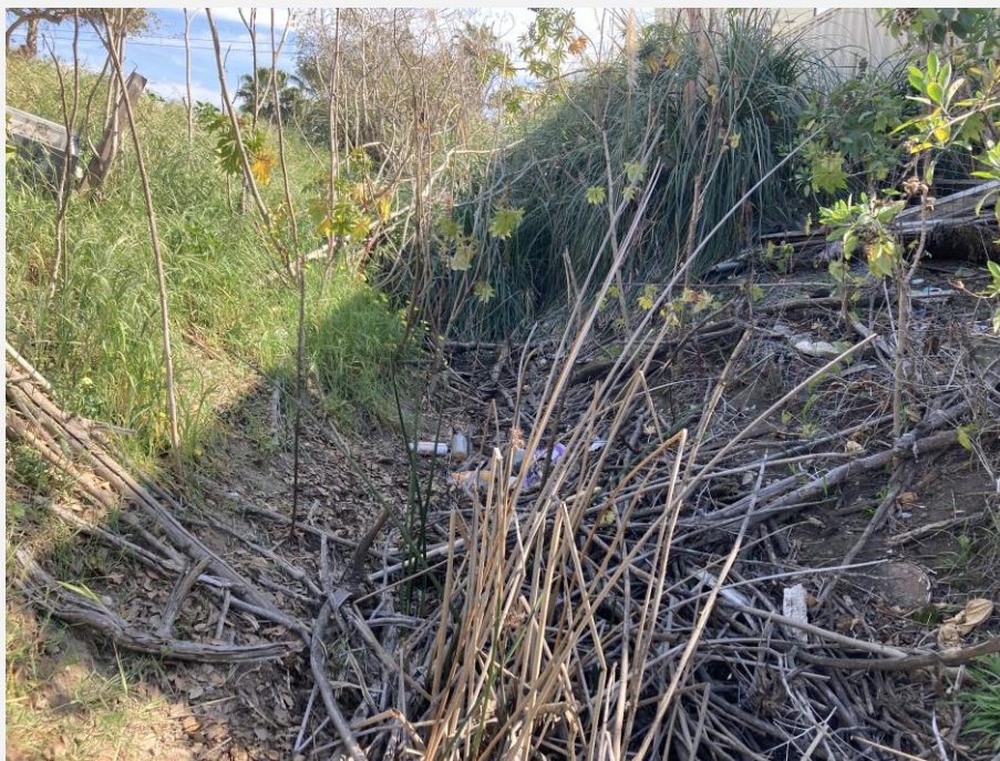
Photo 5. Looking southeast along the storm drain ditch, March 3, 2022
