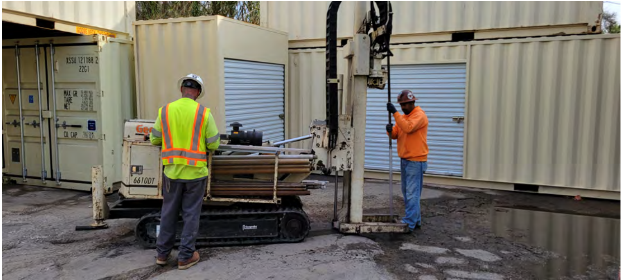
Photo 1. Geoprobe soil sampling at location SB2.
