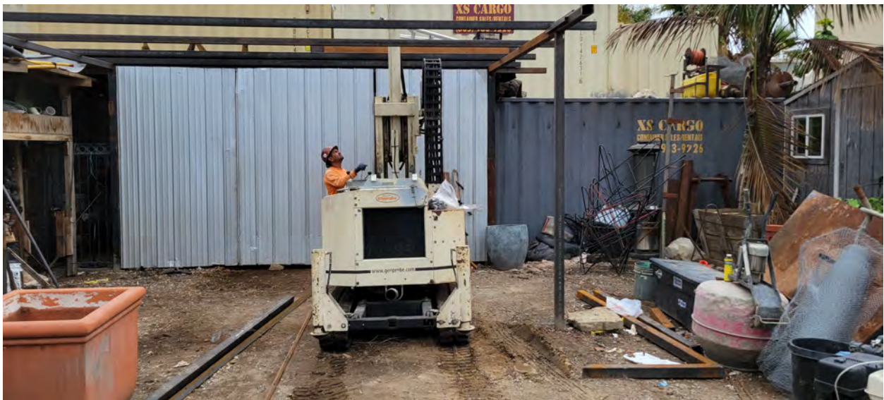
Photo 6. Geoprobe soil sampling at location SB15.
