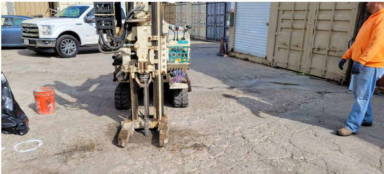
Photo 4. Geoprobe soil sampling at location SB8.
