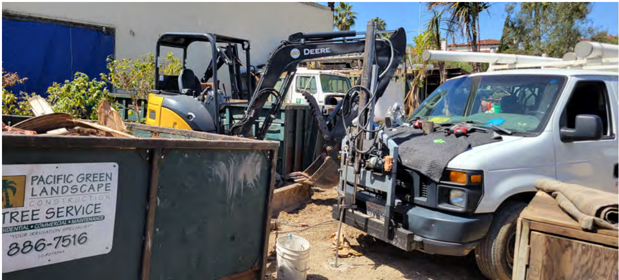
Photo 15. Soil vapor sampling at location SV8.
