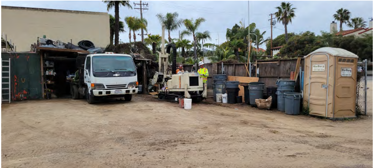
Photo 5. Geoprobe soil sampling at location SB14.
