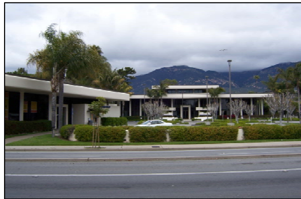
The majority of this development on the north side of State Street is set back from the street, allowing for mountain views across the site.
