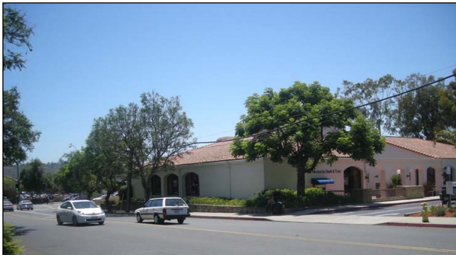
View of entrance to rear parking lot from Hope Avenue.
