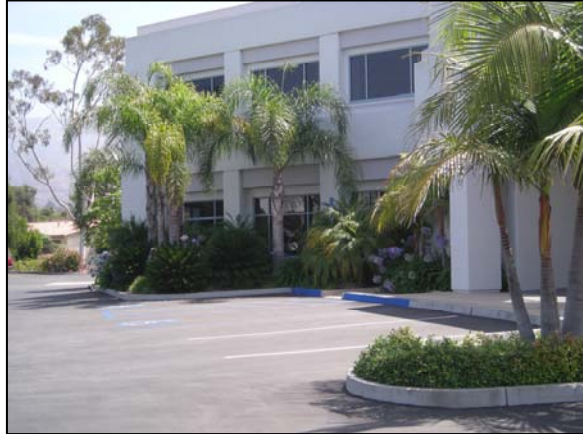
Parking lot landscaping provides greenery and visual texture for an Upper State Street office building.
