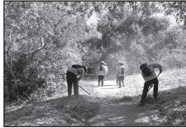
Crew works on a fire access road in Honda Valley Park
