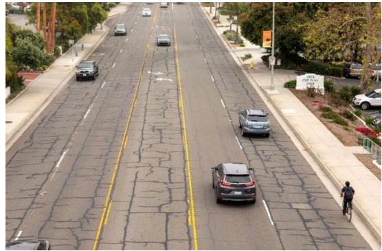
Existing Conditions along Cliff Drive
