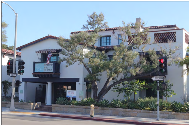
800 Santa Barbara Street
