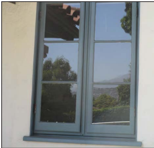
After: The same wood casement window after restoration.
