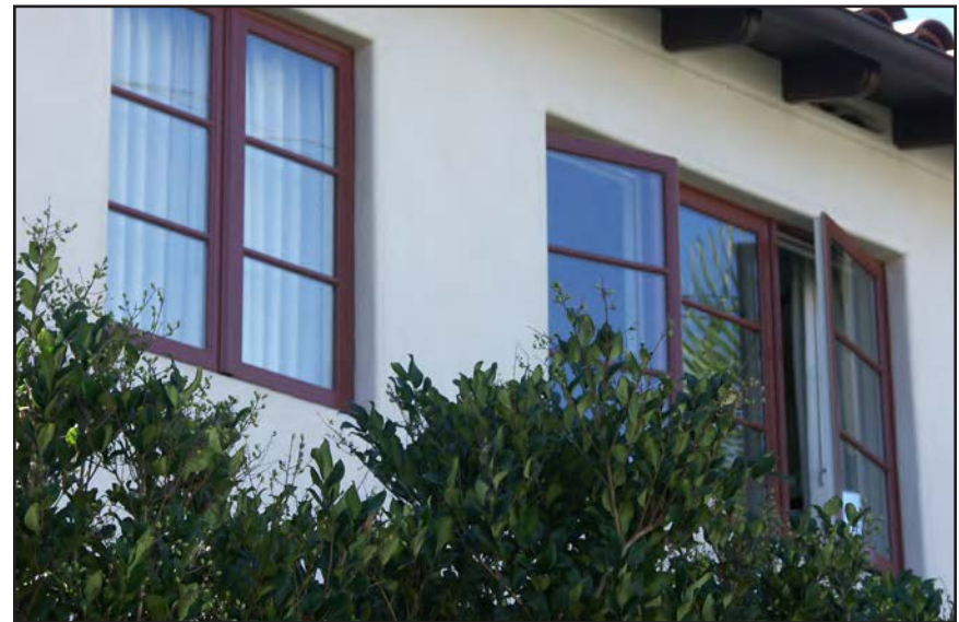
Casement windows with three horizontal true divided lights that are recessed into the stucco façade with no trim.
