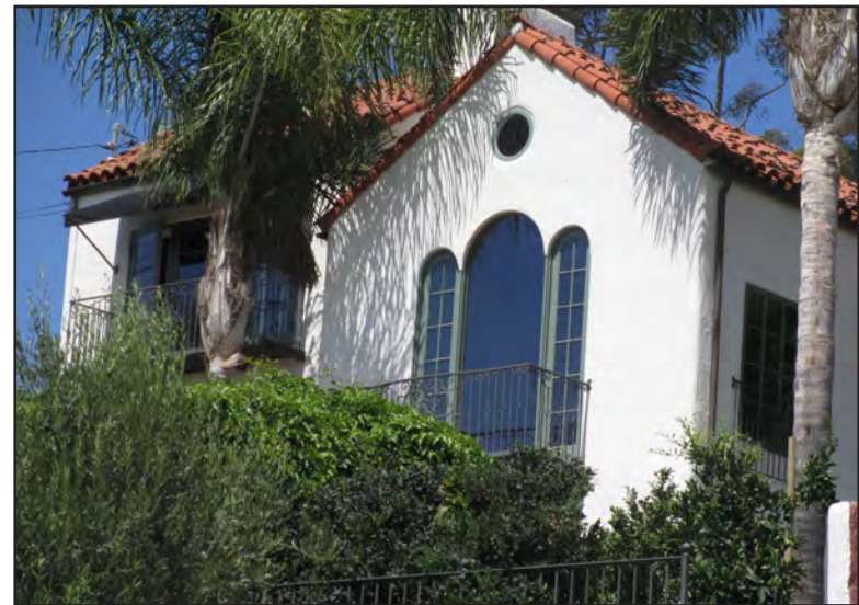
The Spanish Colonial Revival fixed window with sidelights is the centerpiece of the façade and it has been well maintained.
