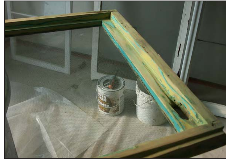
This original casement sash has been removed from the frame and is being restored before being repainted and installed.
