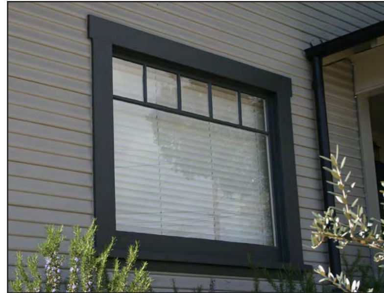
Maintaining the original materials and design of historic windows contributes to the architectural integrity of the structure.
