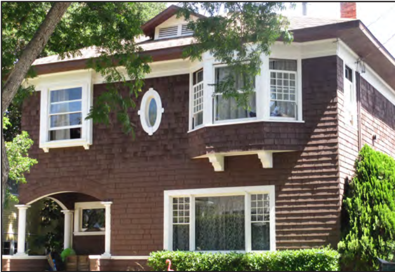
The second floor windows show the top sash of the double hung windows open, allowing a natural cool ventilation through the house.
