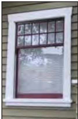
12 over one single-hung wood window with original wood trim with Ogee lugs on upper sash
