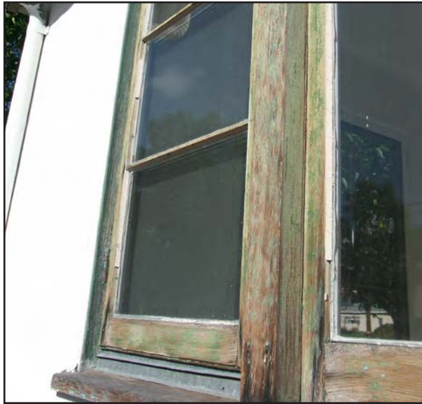
Before: This is an image of a wood window prior to restoration.
