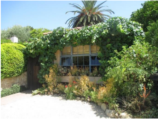
El Caserio, 924 Garden St, Studio "A" constructed in 1930 for violin player, John Vhay. 1948, 1950, 1953 alterations by Lutah Maria Riggs
