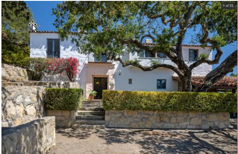
903 Arbolado Road was designed by Vhay in 1922 as her home. Photo taken by Nicole Hernandez, 2022
