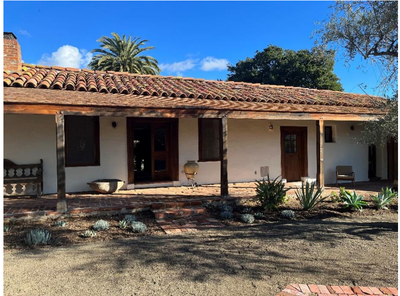
835 Laguna, Ramirez Adobe restored by Vhay. Photo taken by Nicole Hernandez on December 7, 2022
