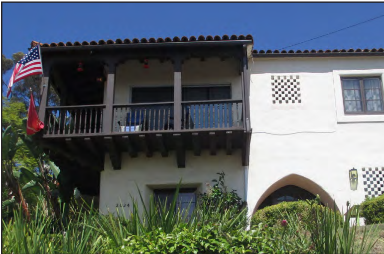
The covered balcony has heavy, wood brackets, on the underside, heavy square posts with brackets and wood balusters.
