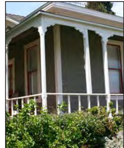
This Folk Victorian building has square posts with decorative brackets with square wood balusters in the balustrade surrounding the porch.
