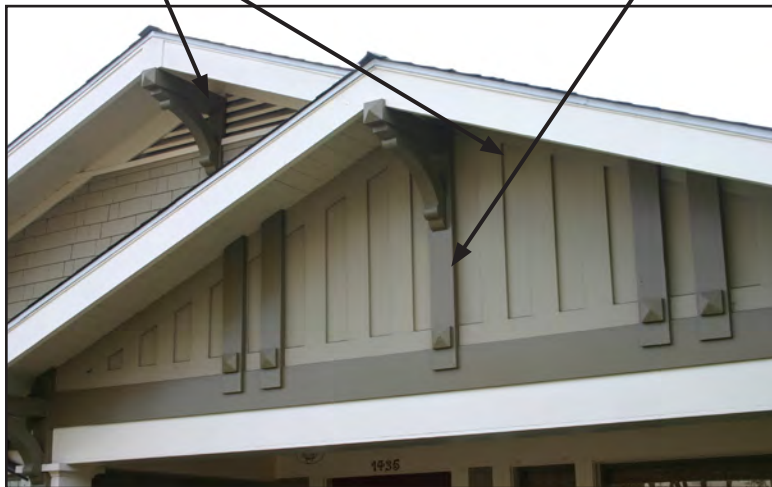
Brackets with exposed rafter tails are typical features of Arts and Crafts bungalows.
