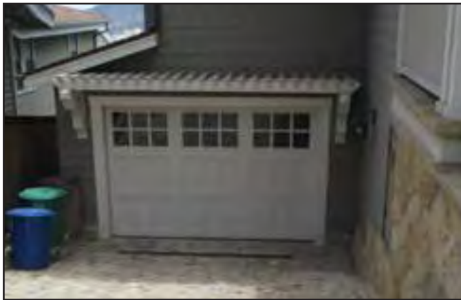
Driveways in historic neighborhoods run down the side of the structure to a simple garage. The garage door design of divided light windows over recessed wood panels successfully reflects the architecture of the neighborhood.
