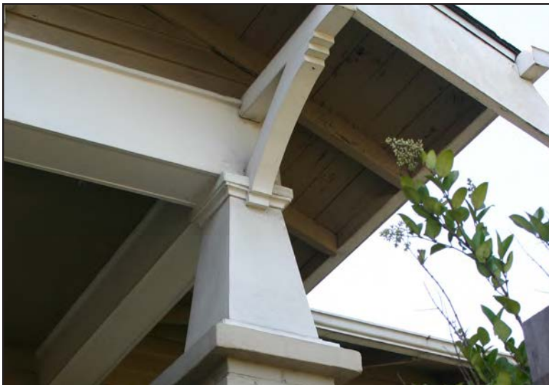
The tapered wood posts on top of a brick pier is a signature feature of a Craftsman style porch.
