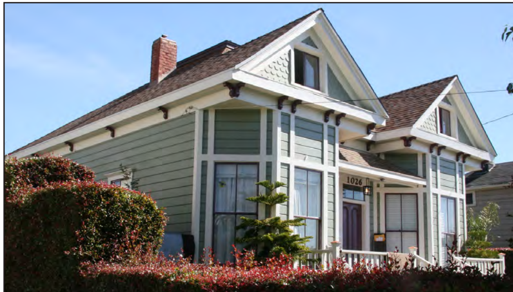
The Stick style residence in the Lower West Side of Santa Barbara expresses its unique decoration with vertical boards dividing the wall, brackets under the overhanging eaves, a transom over the solid paneled wood door and long, two-over-two, double-hung wood windows.
