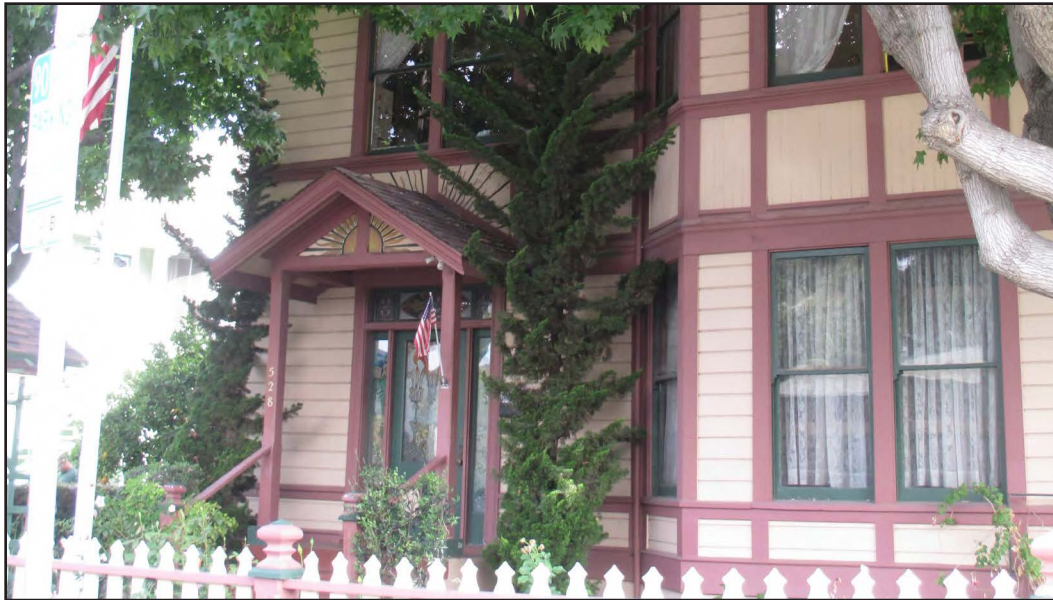
A Stick style house on Brinkerhoff Avenue features horizontal and vertical bands raised from the wood weatherboards for emphasis.
