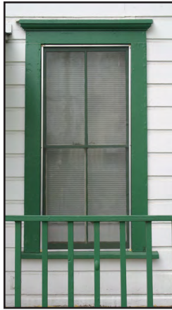
2 over 2 double-hung wood window with original wood trim
