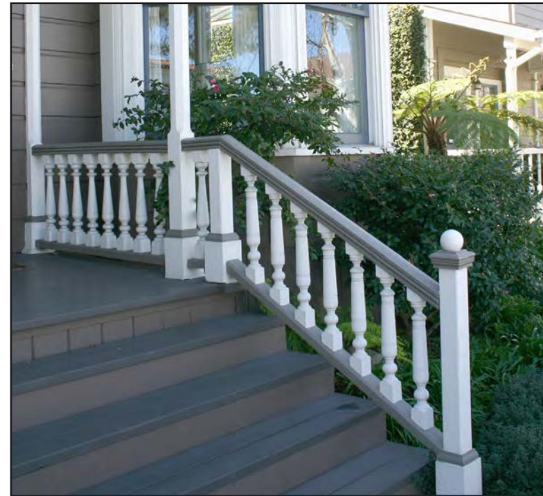
The Victorian era Queen Anne building features wood steps and porch flooring, turned balusters, and chamfered posts with brackets.
