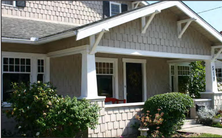
This Craftsman has tapered, square posts with decorative brackets under the eaves, with a low wall finished in the same wood shingles as the house, rather than a railing.
