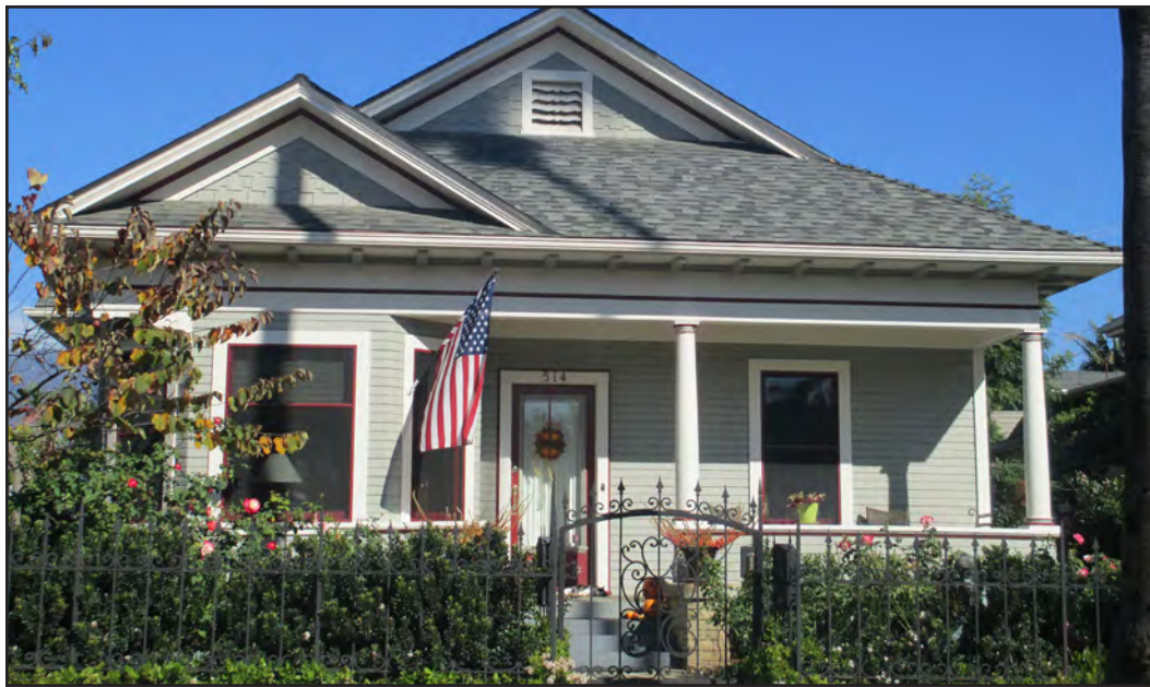
The Queen Anne Free Classic in the Brinkerhoff Landmark District has simple lines at the cornice and simple brackets under the wide overhanging eaves.
