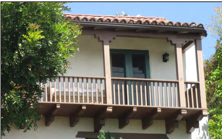
This Spanish Colonial Revival porch features simple, square posts and square balusters on the balustrade with heavy beams under the porch.
