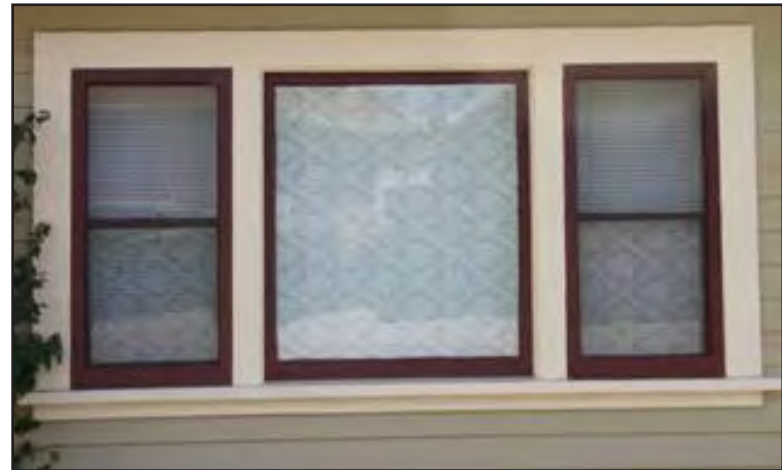
Many Santa Barbara Historic Homes feature a triptych in the center front window with a large window in the center with double hung windows on either side, all in the same opening.
