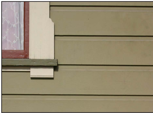
Shiplap (drop lap) siding before and after restoration.
