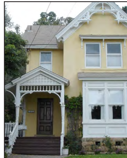
This Gothic Revival style Victorian house features turned columns with decorative brackets and turned balusters on the balustrade.
