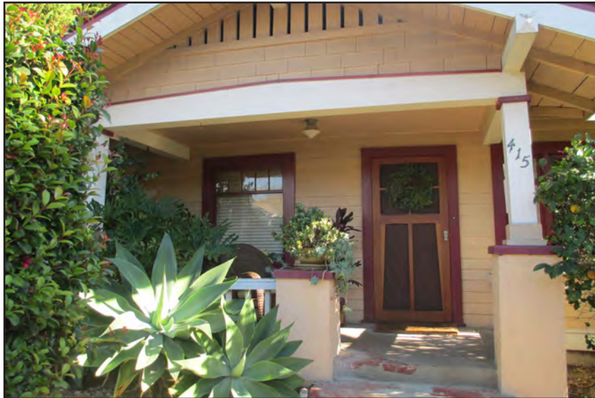
A Craftsman bungalow in West Downtown features shingle siding under in the porch gable and wood siding on the main walls of the house. Notice the large, simple rafter tail under the porch eave and the divided lights of the upper sash of the window.
