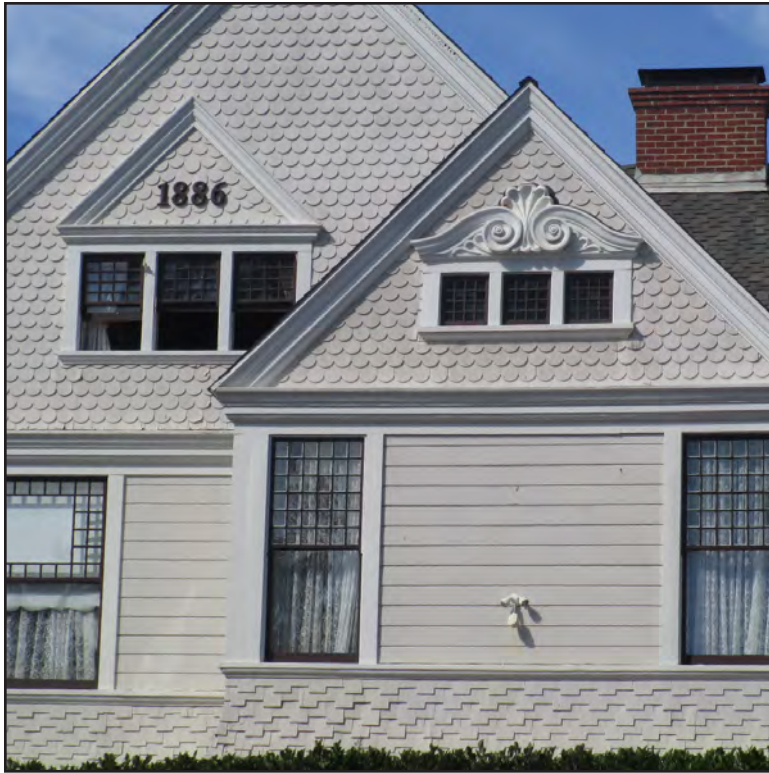
The house features fish scale wood shingles in the gable end combined with shiplap siding and squared shingles on the body of the house.
