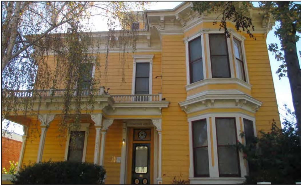
Constructed in 1871-72, this Italianate house on Chapala Street, designed by Architect and Mayor Peter Barber, features paired brackets under the eaves, elongated one-over-one, double hung windows, square porch posts with beveled corners and an ornate front door.
