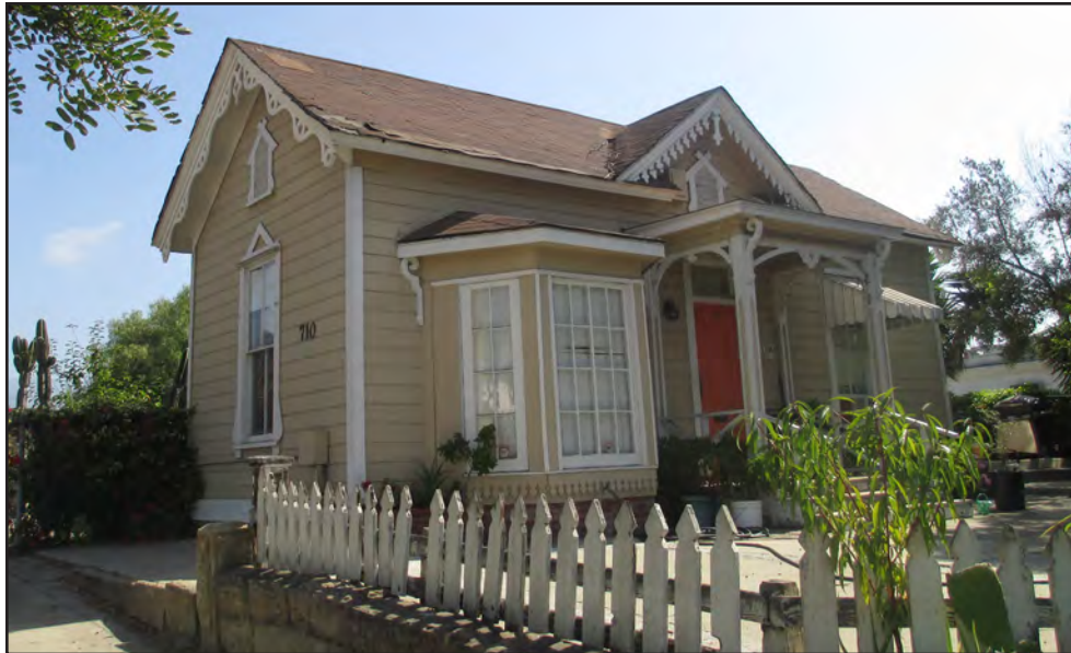
In downtown Santa Barbara a Gothic Revival house has intricate woodwork in the steeply pitched gables, wood cut-outs placed over the rectangular window so that it appears to be pointed and a character-defining bay window
