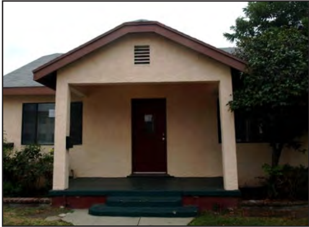
Before: The wood sided Craftsman style bungalow was inappropriately covered with stucco. Photo from the eastsidela.com web site.
