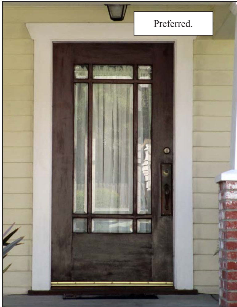
This solid wood door has muntins dividing the glass that adds a decorative element to the door and enhances the entrance.
