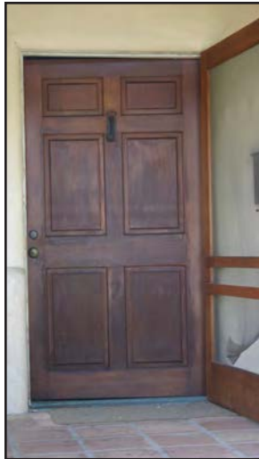
Spanish Colonial Revival six panel solid wood door inset in the stucco with no trim and appropriate wood screen door.
