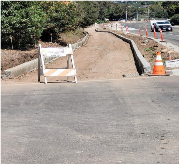
Looking north along Las Positas Road, at the Richelle Street Intersection. Curbs installed, path at final grade and ready to be paved with asphalt concrete on an aggregate base.
