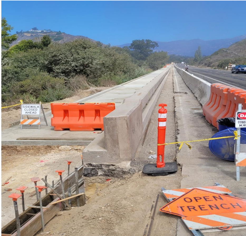
Figure 1: A photo of the concrete path with safety barrier wall along Las Positas Road
