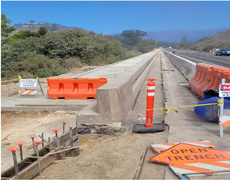
Path under construction on the lower portion of Las Positas Road
