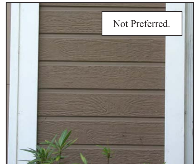
The vinyl siding with faux wood grain appears fake as most wood siding is sanded to a smooth surface (See photograph on page 28) If using an alternative siding like a cement fiber to imitate wood, use the smooth finish for a more authentic appearance.
