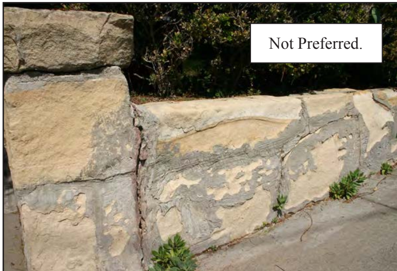
Poor maintenance and improper repointing can damage stone walls.
