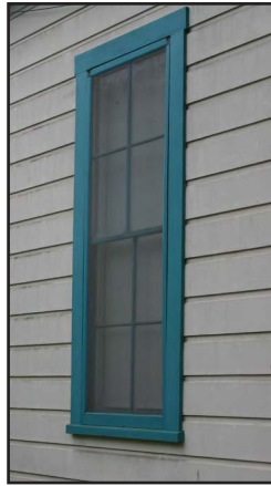
4 over 4 double-hung wood window with original wood trim
