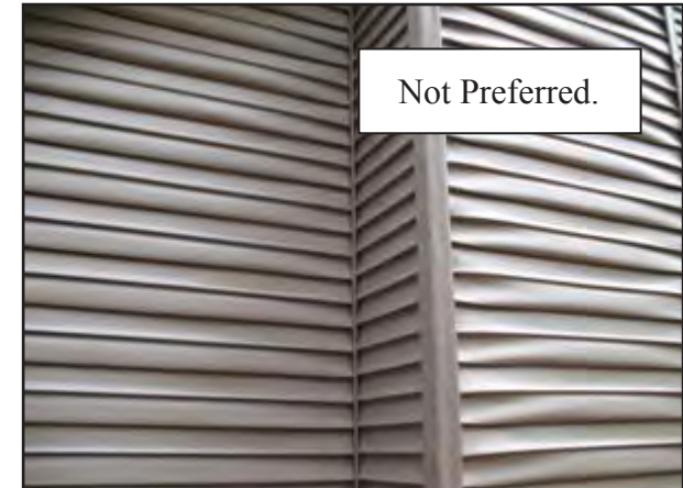
This artificial siding warped from sun exposure.
