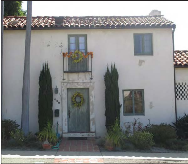
Using true stucco rather than a synthetic stucco is recommended for repairing stucco on Santa Barbara historic resources.
