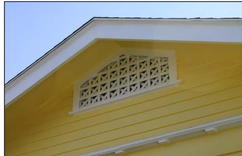
The Craftsman home features original, decorative venting in the gable that helps vent the attic space.
