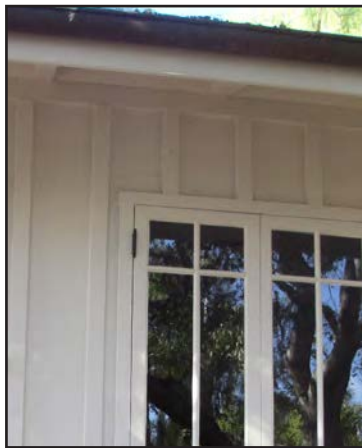
Board-and-batten siding on a Craftsman style home.
