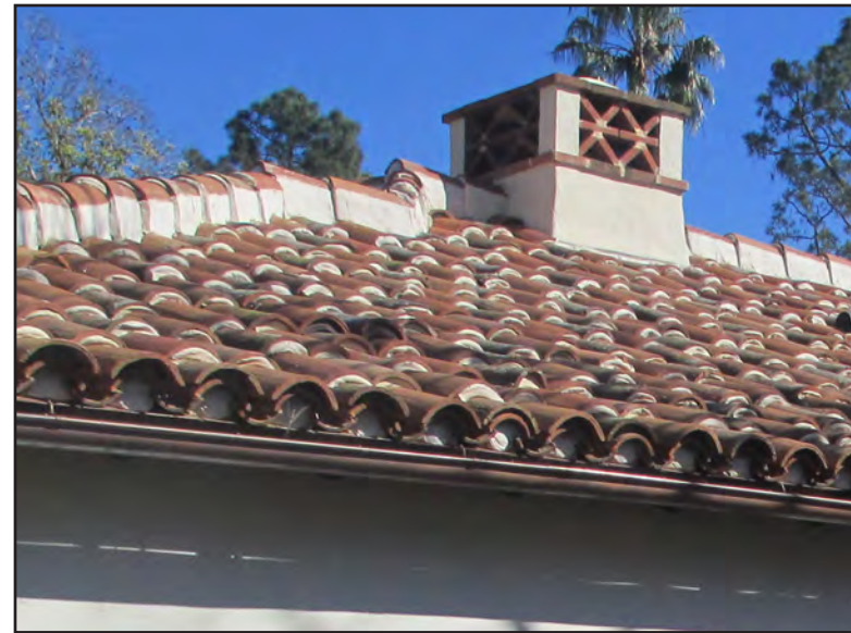
The starter courses of two-piece cap and pan terra-cotta roofs in Santa Barbara are double tiled.
