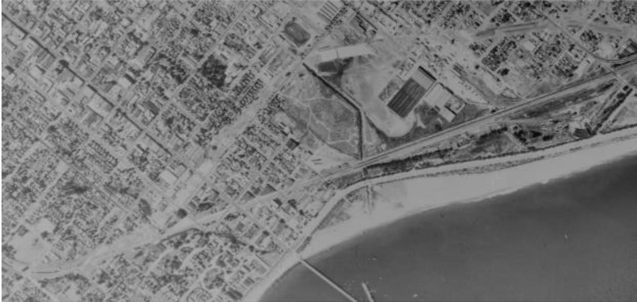
Figure 23. Aerial photograph, showing blocks cleared for construction of U.S. Highway 101/State Highway 2 (1947). Source: Flight GS-EM, Frame 6-112, Harry Tubis, Inc., UCSB FrameFinder.
