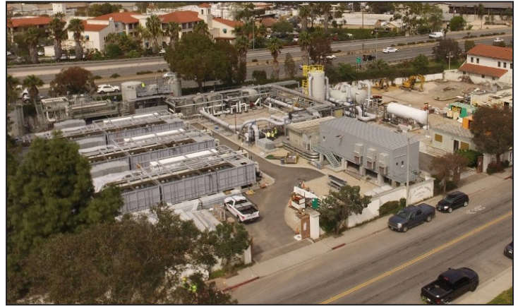
Aerial image of Charles E. Meyer Desalination Plant March 2017
