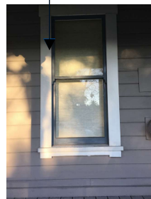
FRONT WINDOW - ORIGINAL CONSTRUCTION
