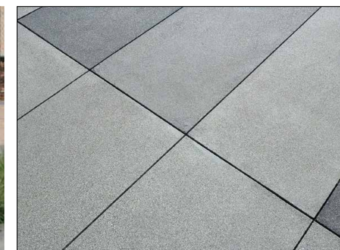
CONCRETE WITH SCORING
