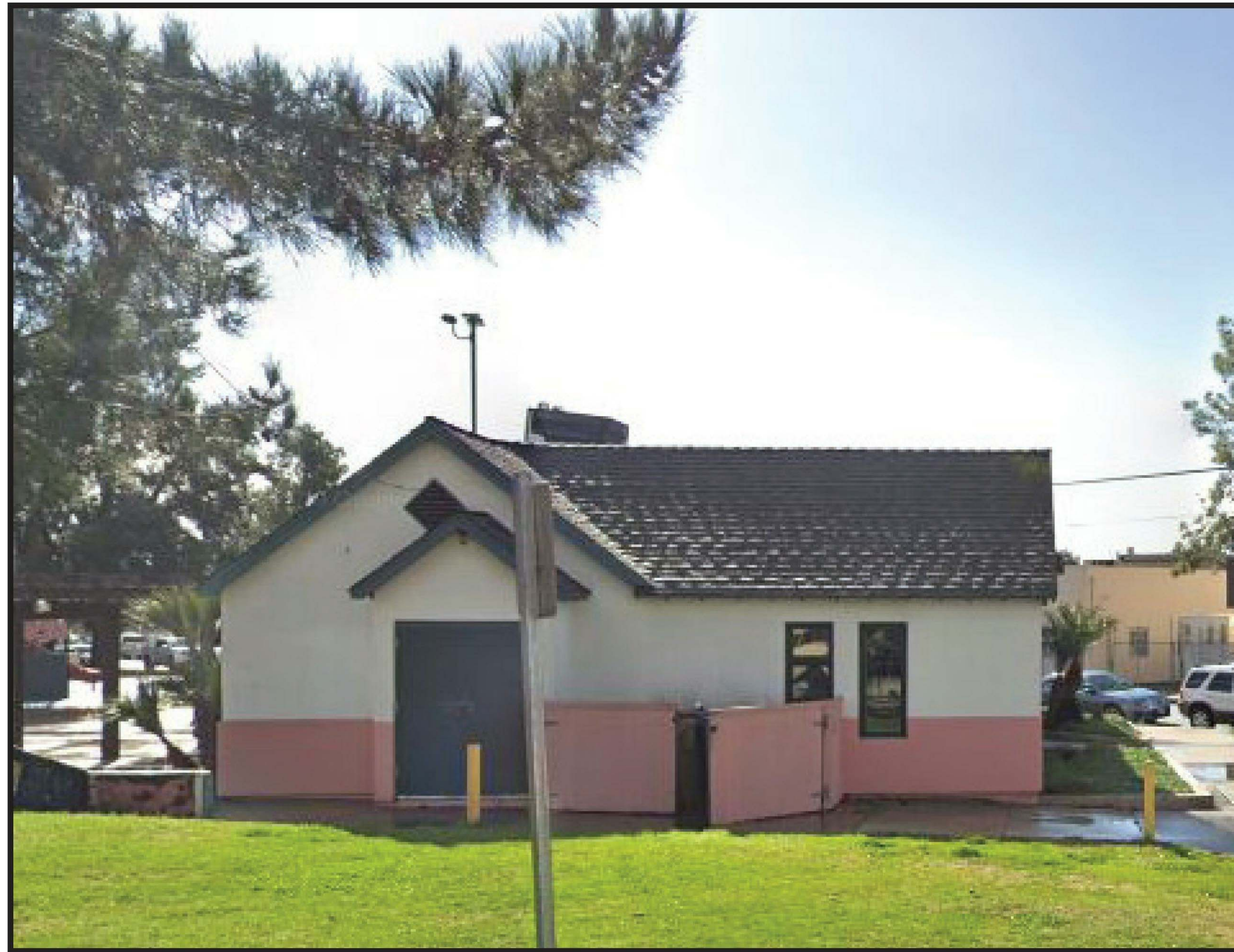
EXISTING WELCOME HOUSE NORTH ELEVATION
