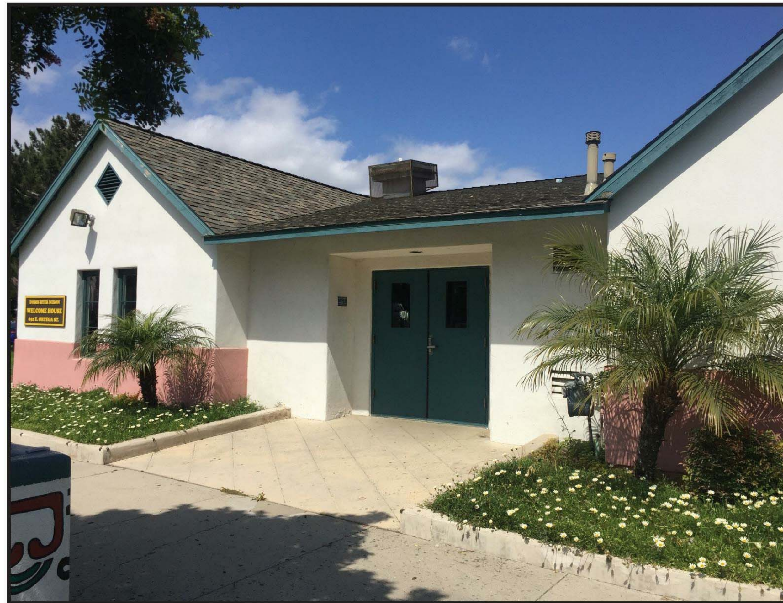
EXISTING WELCOME HOUSE MAIN ENTRANCE
